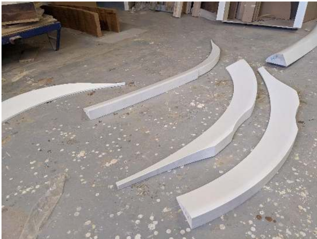
- Ceiling parts first layer of lacquer and rough sanding
