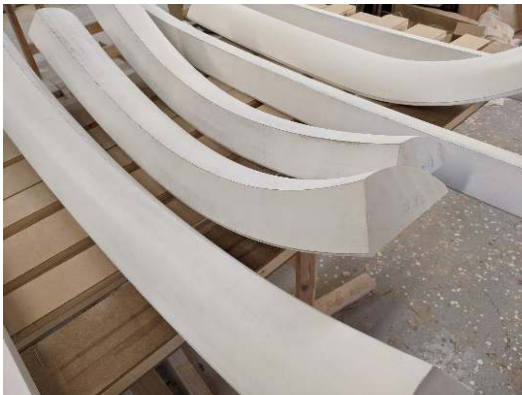
- balcony parts first layer of lacquer and rough sanding
